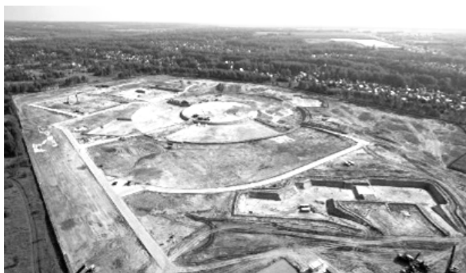
Fig. 1. Construction site of the Synchrotron Radiation Facility SKIF (as of summer 2022).
